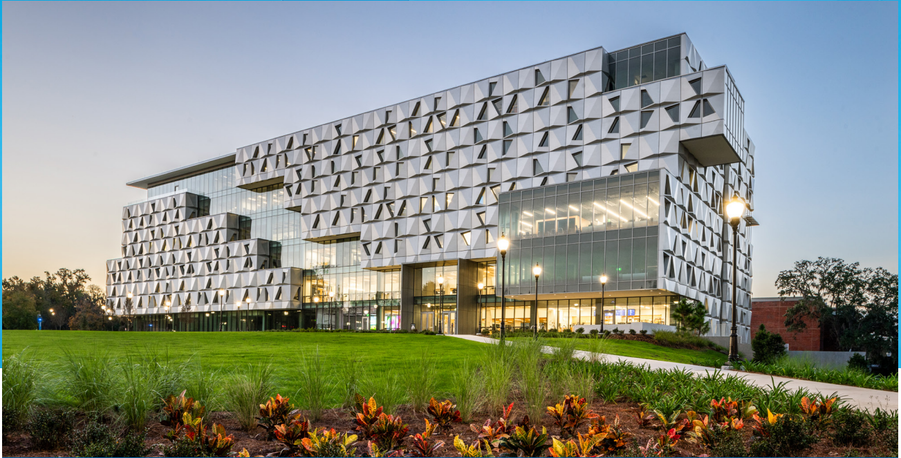
KENPAT: The stunning geometric façade of Malachowsky Hall for Data Science and Information Technology at The University of Florida in Gainesville, Florida. N-RG Cladding served as the design-assist partner for the state-of-the-art, 263,000-square-foot, award-winning facility. ABC National Excellence in Construction® Award Winner
