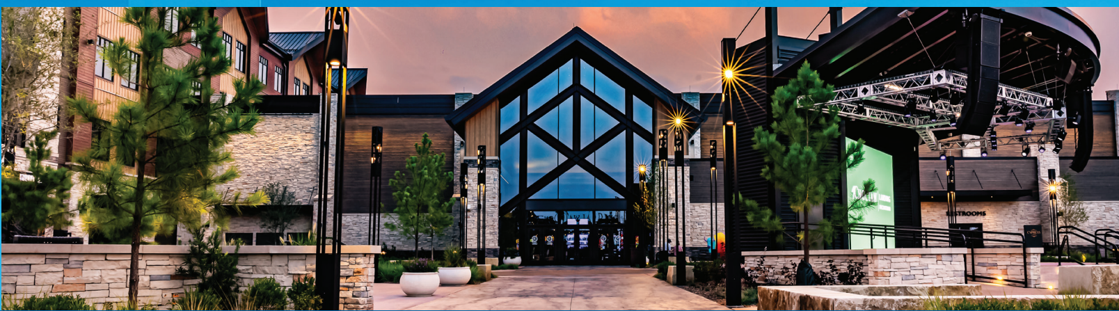
Manhattan Construction Co.: Choctaw Landing is a stunning, new, four-story, 175,000-square-foot entertainment and resort development in Hochatown, Oklahoma. ABC National Excellence in Construction® Award Winner
